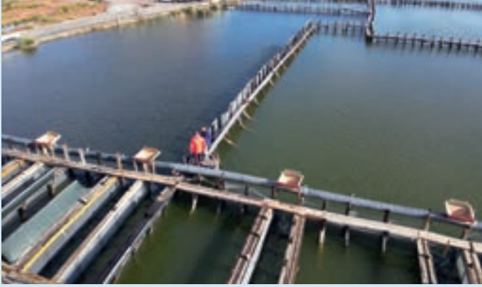
A system of weirs is used to trap fish, mainly mullet, seabass, seabream, and eel, as they migrate from the Köyceğiz lake to the Ionian sea and back.
