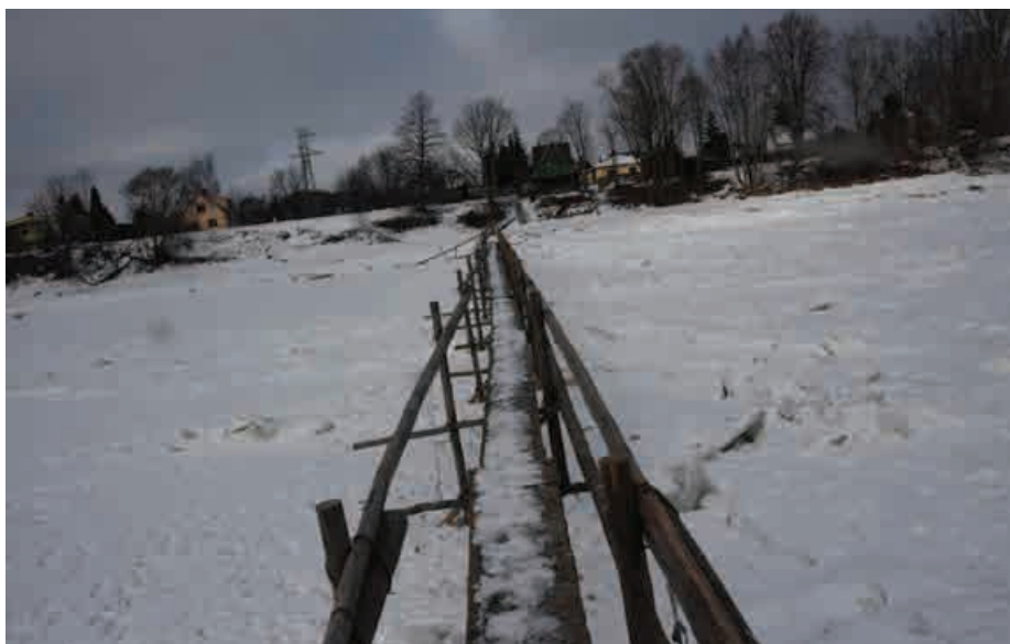
The bridge to which the lamprey traps are attached. Made of wooden stakes tied together with steel wire, the bridge is rebuilt each season.
