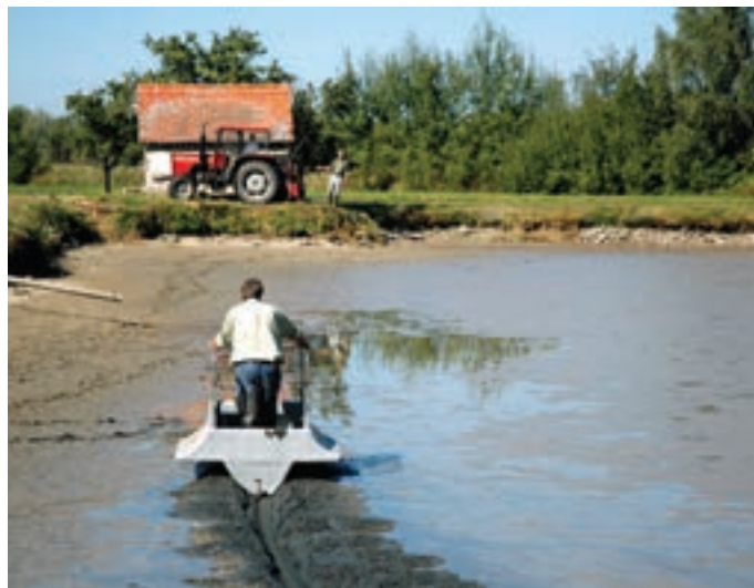
The sediment contains countless microorganisms that release geosmin and 2-methylisoborneol. This is why the sludge should be regularly removed.
