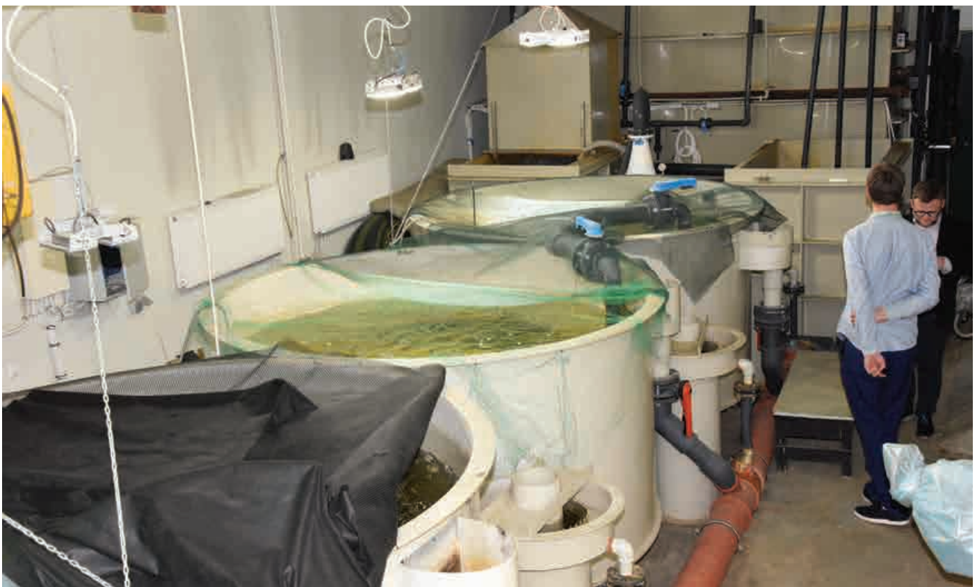
One of the recirculation aquaculture systems at the Aquaculture Centre
